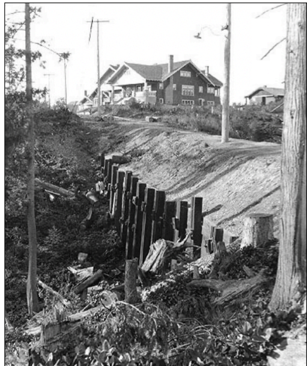
2. NE 62nd Street viewing northwest, 1910.
