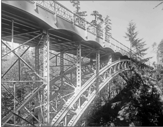
1. 20th Street Bridge, National Historic Register.
